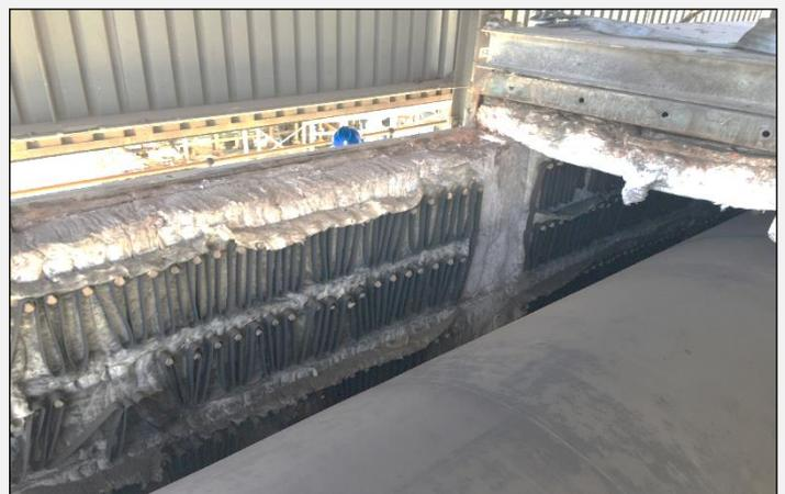
**The cabinet roof must be removed to access elements – estimated down time for inspection and replacement of distorted elements is 20hrs**
