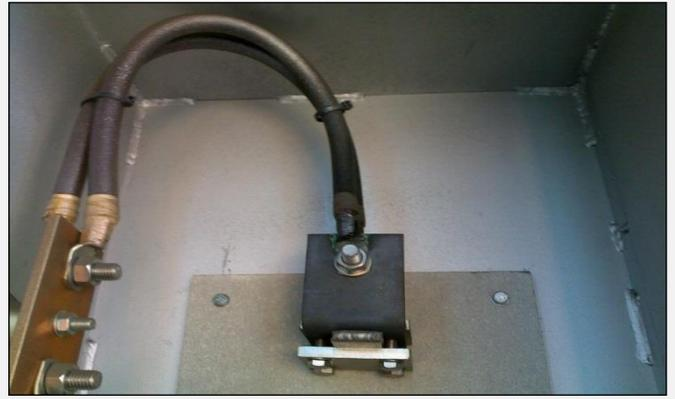
**Electrical connection onto bus bars – the discolouring of the bus bar can be seen**
