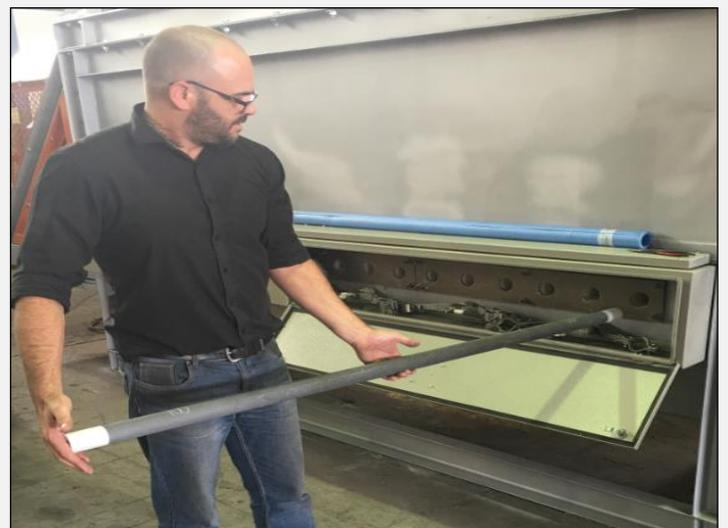
**Installation of SIC element from outside of kiln with no mechanical access required, only electrical isolation required**
