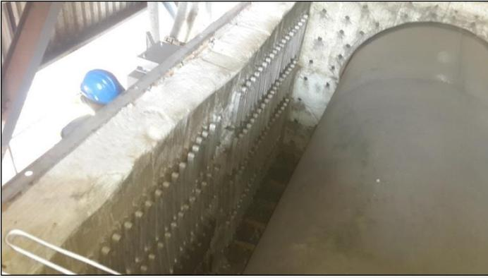
**New replaced strip elements – actual down time to complete repairs 52 hours**
