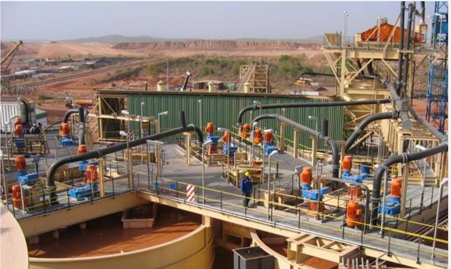
**Carbon-in-pulp plant with two mineral processing separating pumping interstage screens per tank and tanks positioned with the same horizontal elevation**
